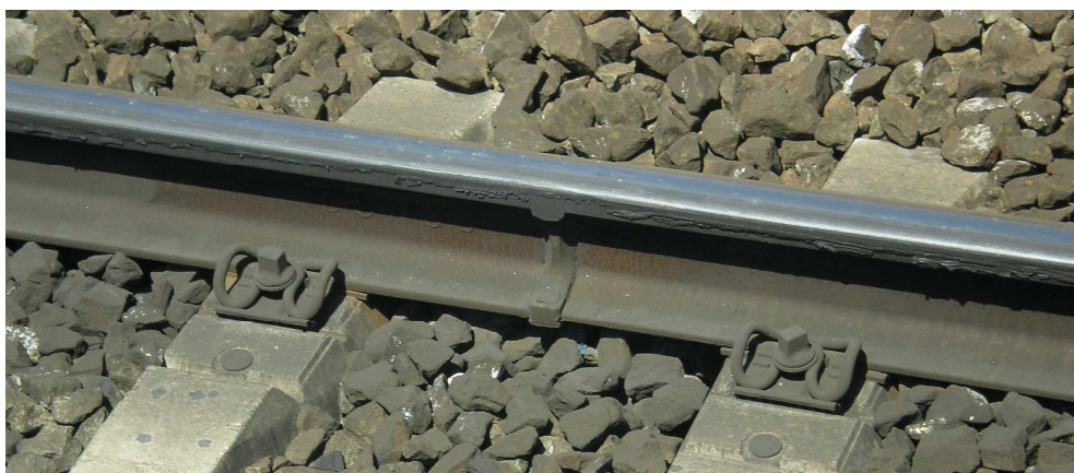
Fig. 1. A typical rail weld in a ballasted track.
