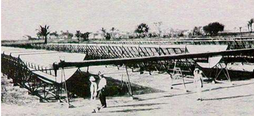
Figure 6. PTC plant designed and build by Frank Shuman in Meadi.
