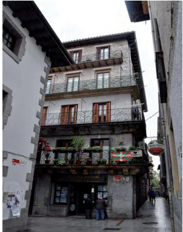
FIGURA A9. 3. FACHADA PRINCIPAL A C/ MAYOR
