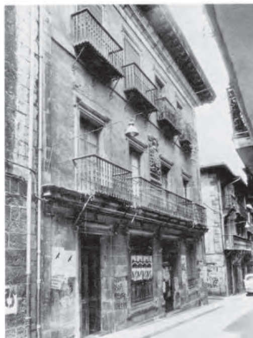
FIGURA A3. 6. 1982, FACHADA PRINCIPAL 2
