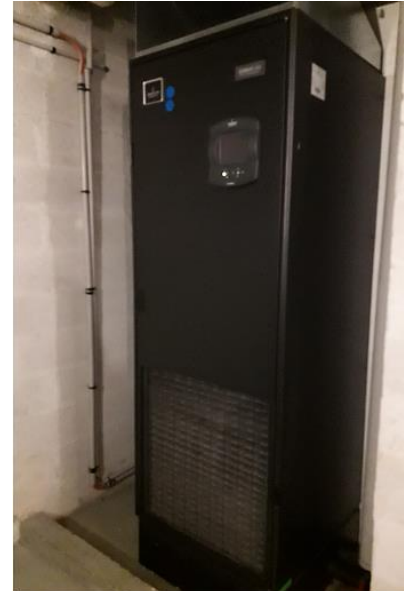
Figure 8: Climatisation Autonome
