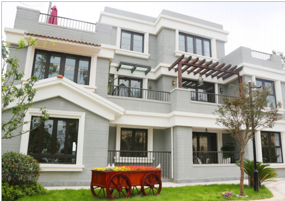
Figure 16: Wujiang 3D Printing Three-storey Villa [73].
