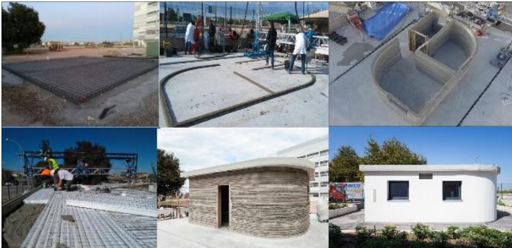
Figure 17: Construction process BE MORE 3D [74]
