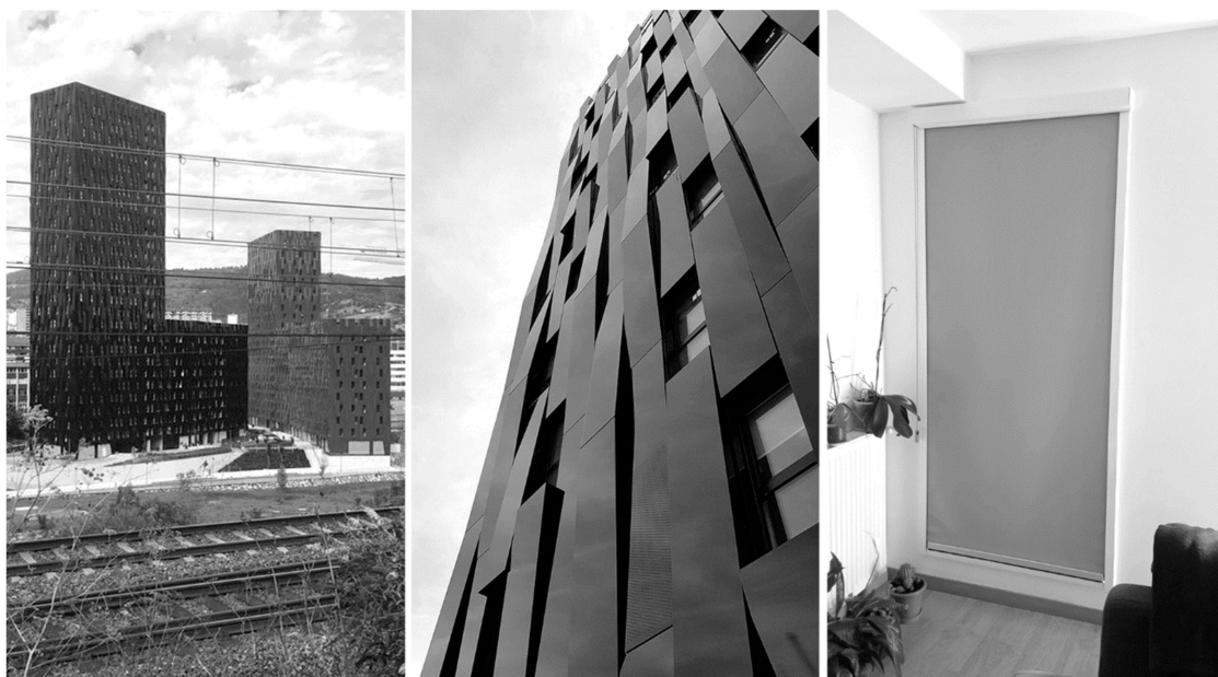
Figure 2. (Left) View of the monitored building. The 2nd tower, still in construction when the photo was taken, can be seen in the background. (Center) Close up of the façade, where the black aluminium façade panels and the size of the windows can be appreciated. (Right) View of the window of a living room, with the interior sunshade. Source: Authors.
