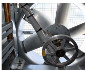
Figure 4. Condensers' fans
