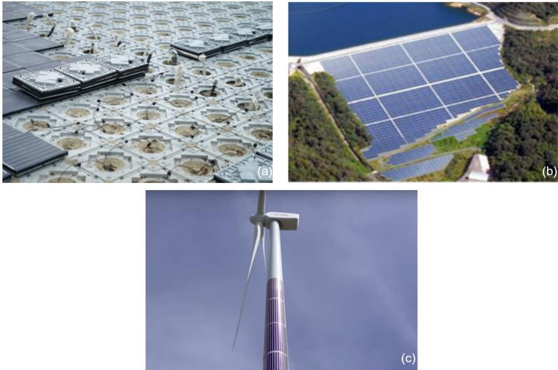
Figure 27. Examples of new integration surfaces: a) PV pavement in Barcelona, Spain (Otero, 2021); b) PV installation in Kotani Dam, Japan (Ioannis et al., 2014); c) PV system trial on a windmill in Spain (Richard, 2019)
