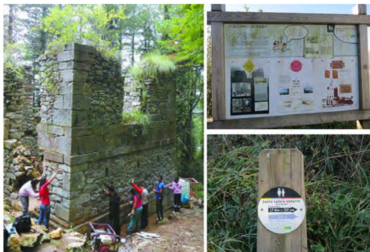
Figure 10: Left: Volunteers performing conservation tasks in the tower of Tolosa. (Arandia, 2011). Right: Current signage in the Santa Lutzia-Uzturre route. (Photographs by the author, 2021)
